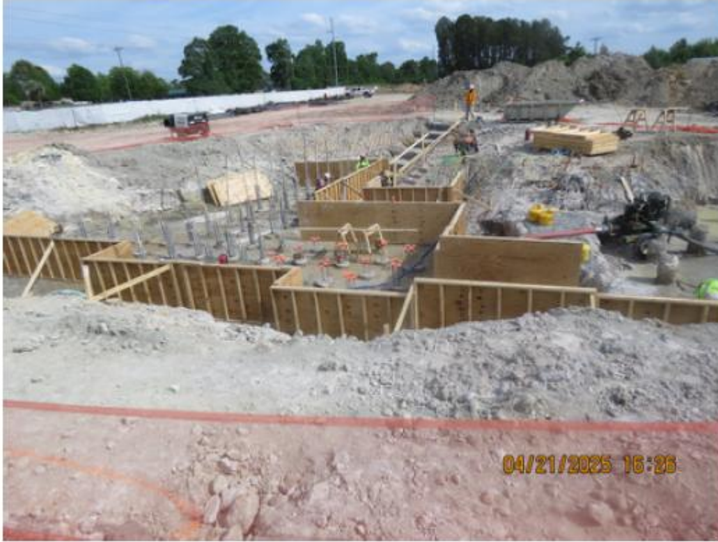
Forming Mat Foundation at Stair 4 & Loading Dock
