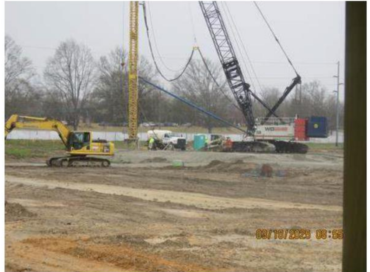
Drilling auger cast piles
