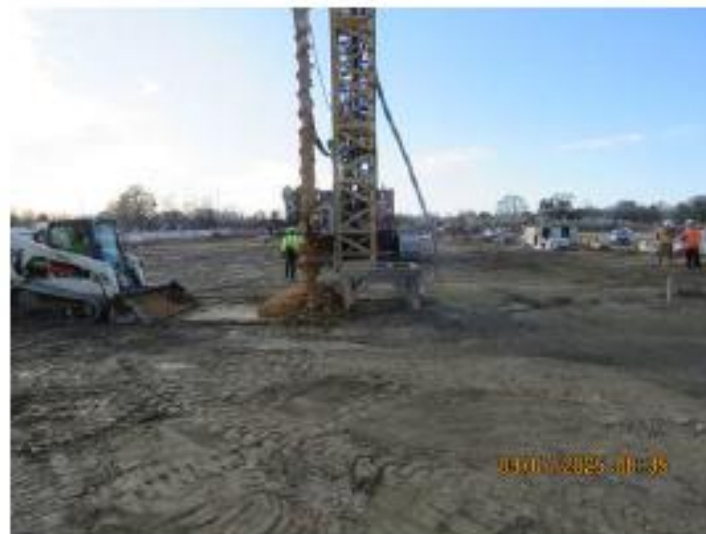
Keller Continuing with Case Piles
