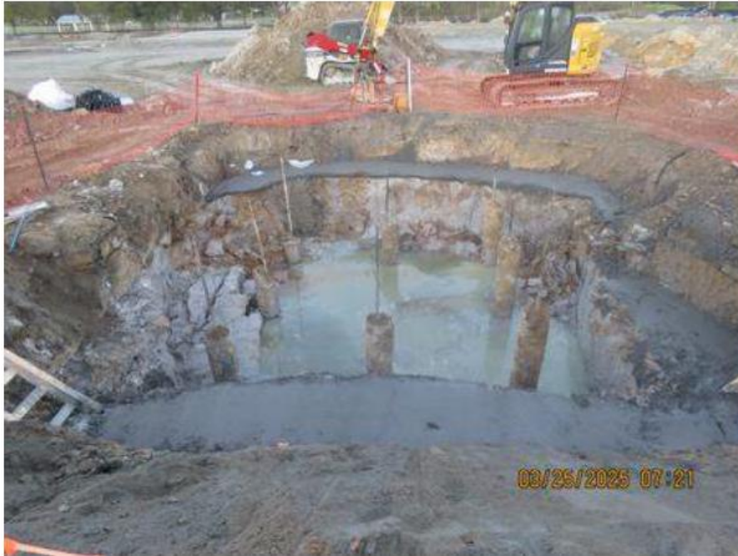
Tower crane foundation excavation and mud mat (water is ground water seepage)
